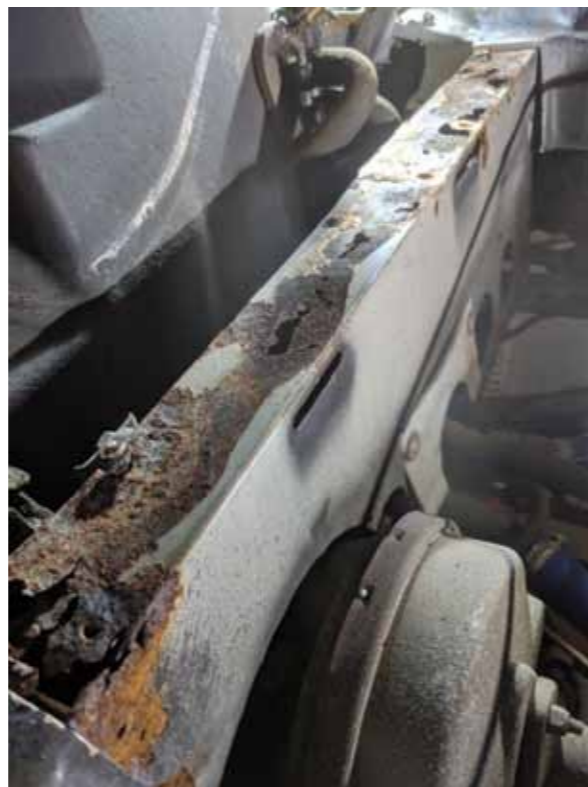
The badly corroded cross member
