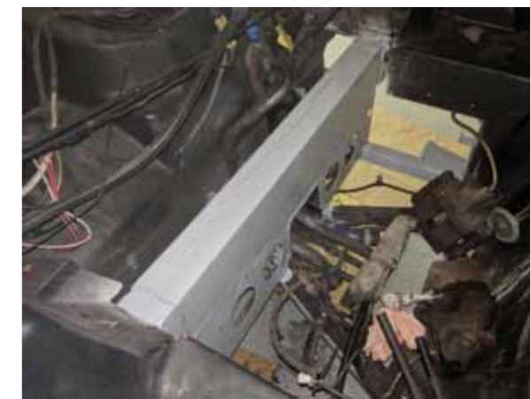
Repaired cross member
